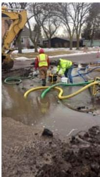
Concrete was removed and excavating was started all while full pressure was still on the main. Three gas-powered trash pumps were used to keep up with the flow until the main was exposed enough to put a repair sleeve on. Finally by 5 p.m. Thursday, the leak was repaired.
