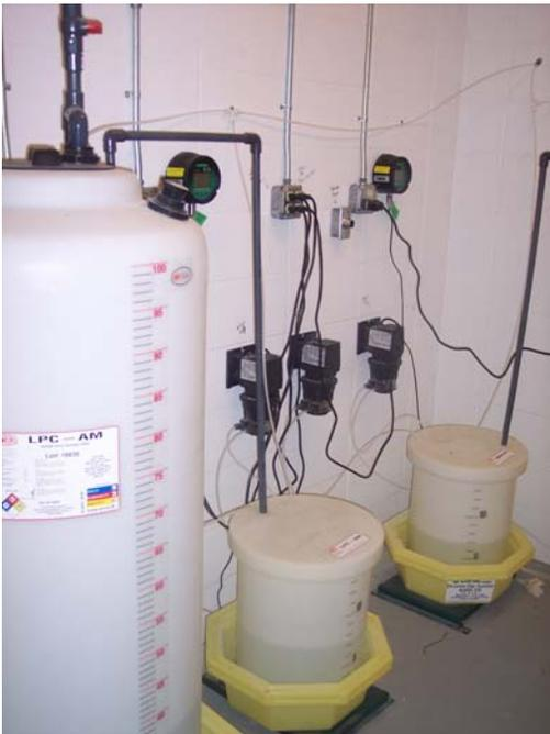
Chemical feed set up for iron and manganese control
