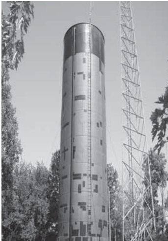
Plattsmouth Standpipe Constructed in 1887
