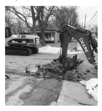
Concrete was removed and excavating was started all while full pressure was still on the main. Three gaspowered trash pumps were used to keep up with the flow until the main was exposed enough to put a repair sleeve on. Finally by 5 p.m. Thursday, the leak was repaired.
