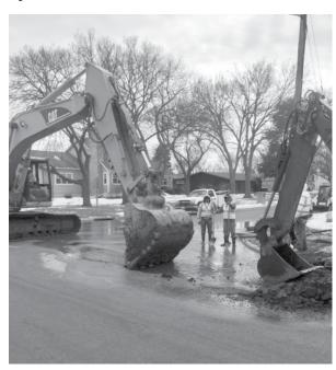
Almost every valve we shut needed to be located under the snow and ice. We had to chisel and torch the ice and rust just to get the lids off. Some valves were under gravel roads that needed to be thawed and dug out as well. Needless to say, at the end of the day, we had closed 14 valves and still had full pressure at the leak site, so we called it a day.
