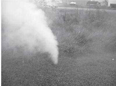
Mostly we find numerous smaller openings into the collection systems such as missing cleanout caps, etc. but they all add up. We have found rain gutters connected to the city sanitary sewer and direct connections between the sanitary and storm sewer systems. With the extremely high costs associated with treatment expansions sewer smoking is very cost effective.
