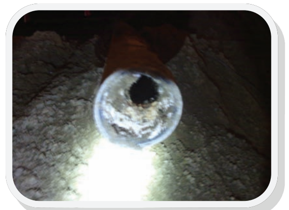
A section of pipe plugged with grease
