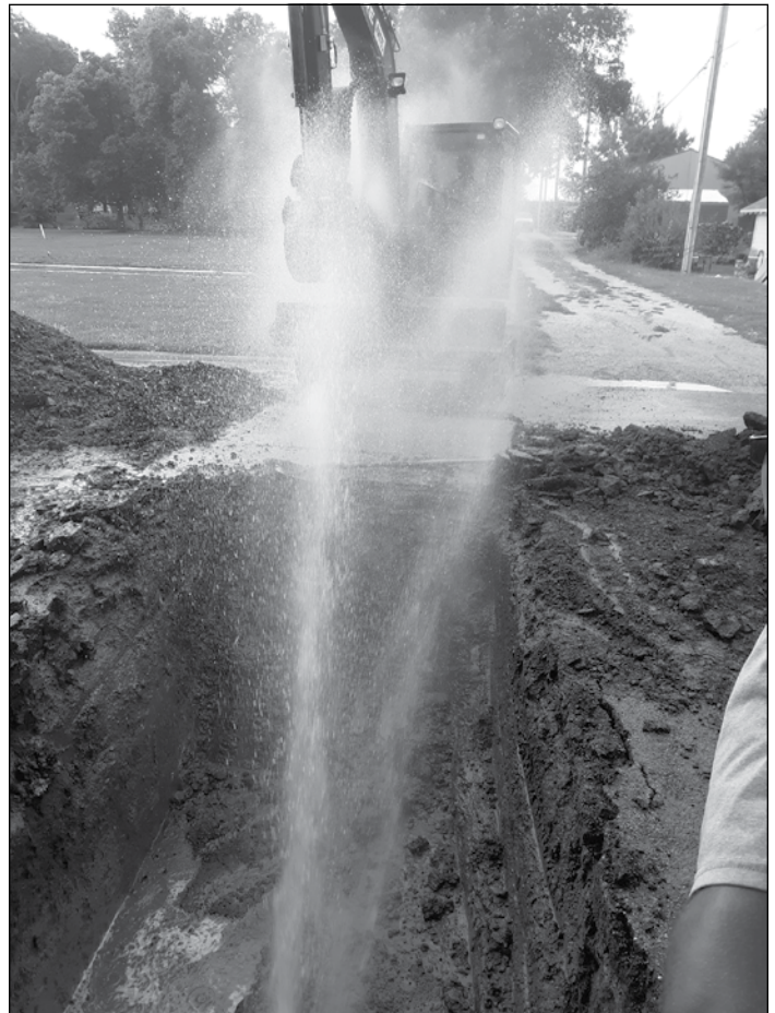
Picture 2: Backhoe getting a bath
